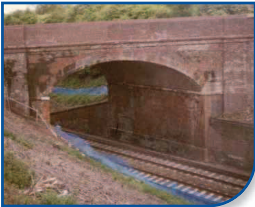
Bridge Abutments London to Brighton Mainline
