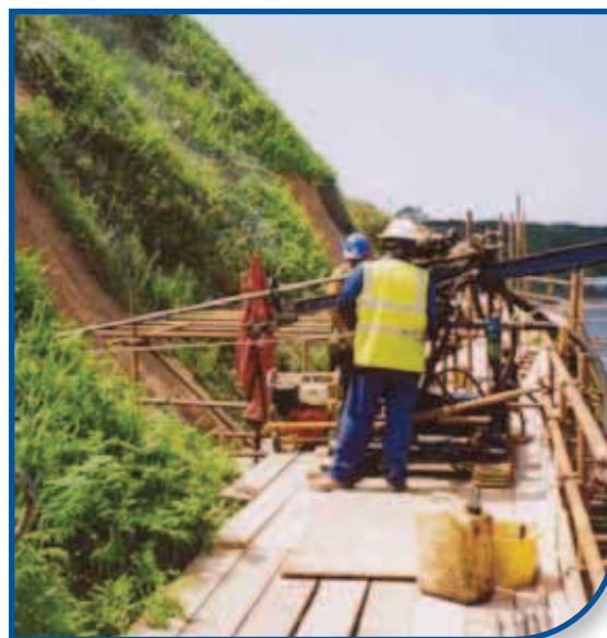
Cliff Stabilisation Nefyn, Gwynedd, North Wales
