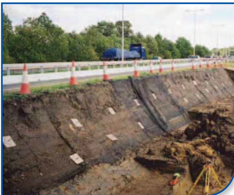
Embankment Stabilisation The A2 at Boughton
