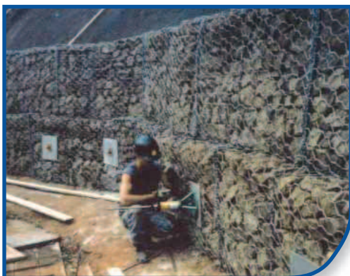
Gabion Baskets Nelson Close, Exeter
