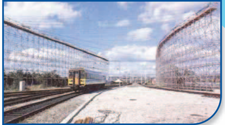
Scaffolding Power lines crossing railway tracks
