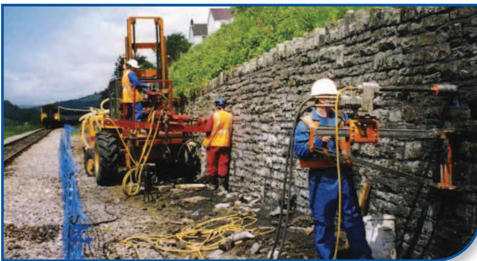
Retaining Walls Merthyr Vale
