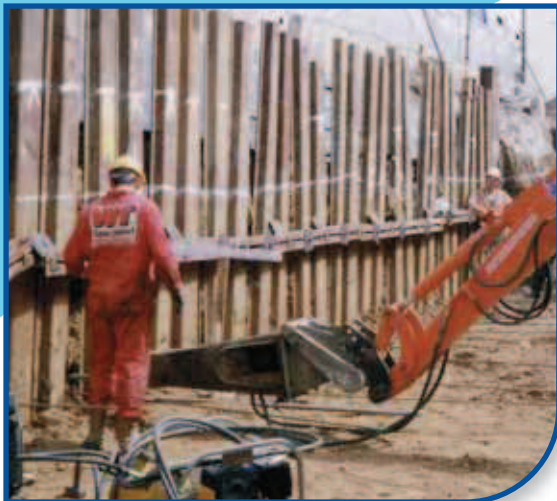
Sheet Piling Docklands Light Railway
